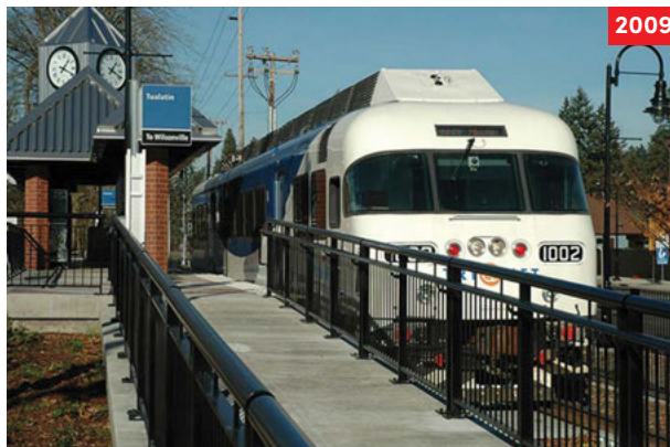
More than 10 years in the making, TriMet's 14.7-mile Westside Express Service Commuter Rail line opens on Feb. 2.
