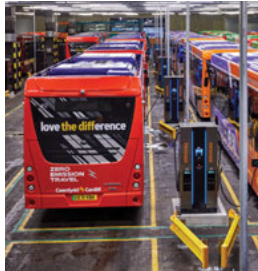
An electric bus being charged.
