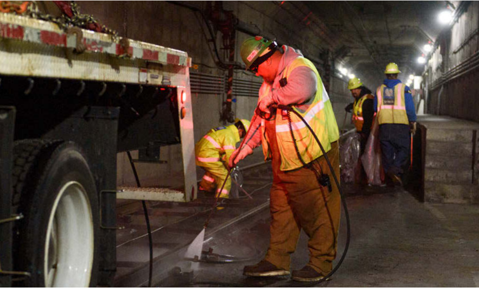
Track crew power washing and removing trash from trackway during Fix It Week night maintenance work.
