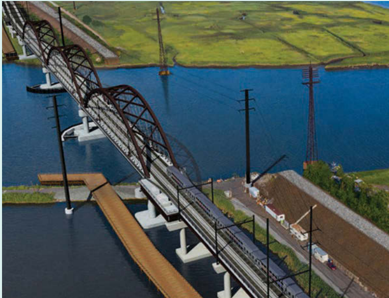
A rendering of the Portal North Bridge project.
