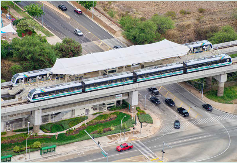
The Honolulu rail system, Skyline, opened for service on June 30.
