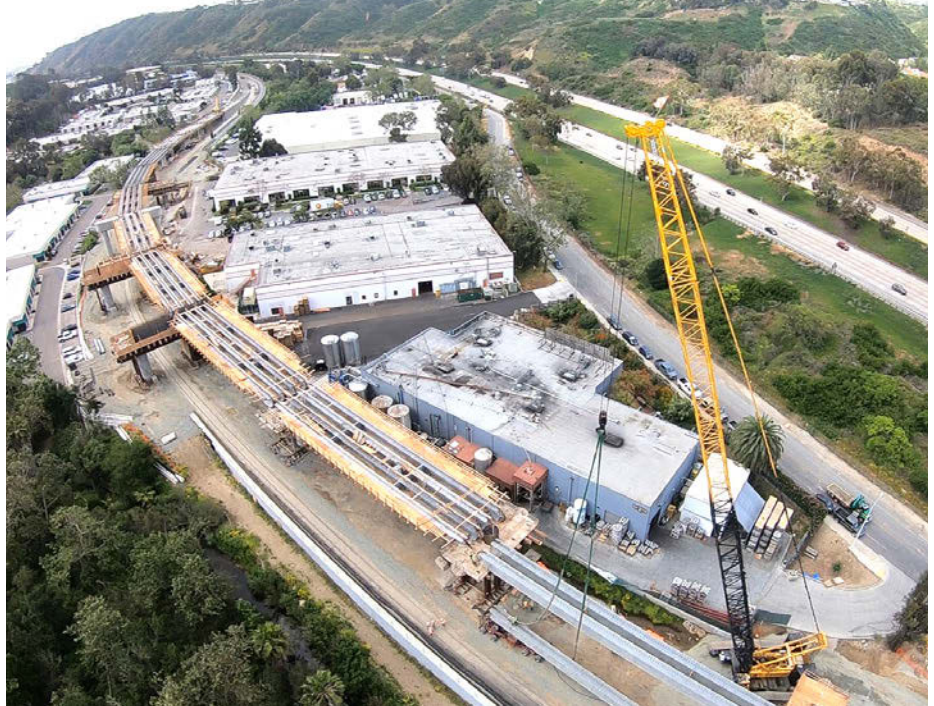
THE MID-COAST Corridor work included 21 bridges.
