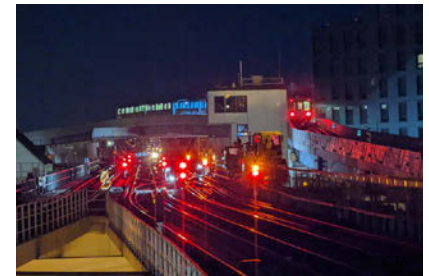
THE BYPASS allows Brown Line trains to go over Red and Purple trains, increasing capacity and reducing delays.
