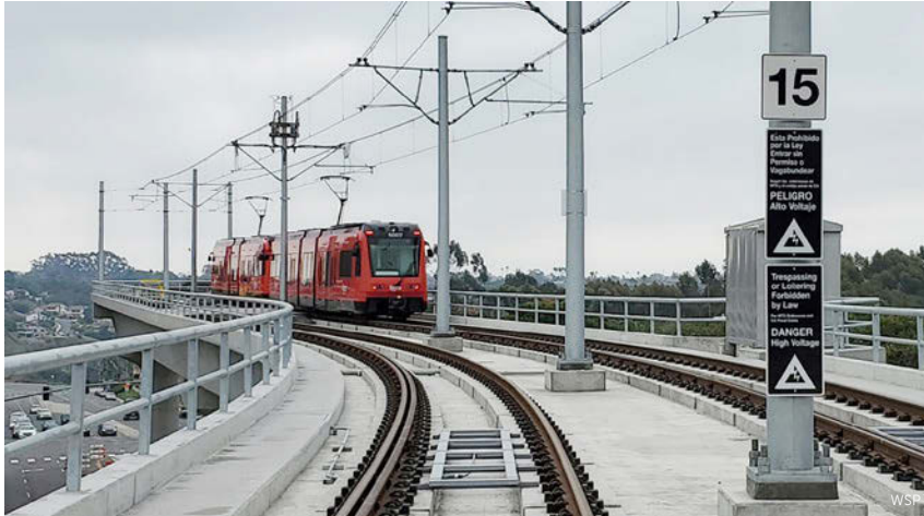
THE MID-COAST Extension included constructing 11 miles of double track infrastructure.
