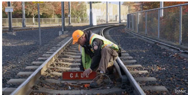
A TRIMET track inspector sets up a call board at one end of a work zone. Call boards are one safety component utilized when working on or near live track.
