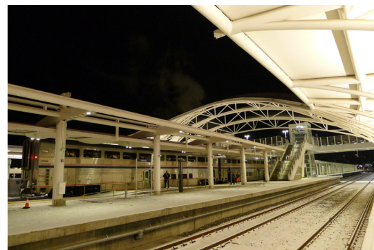
The platform canopy behind Denver Union Station in November 2014. Source: Rochelle Carpenter, T4America
